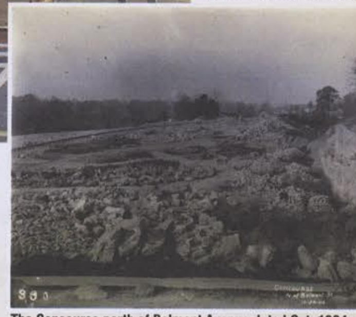
The Concourse north of Belmont Avenue dated Oct. 1904.
